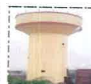
ELEVATED STORAGE RESERVIOR
